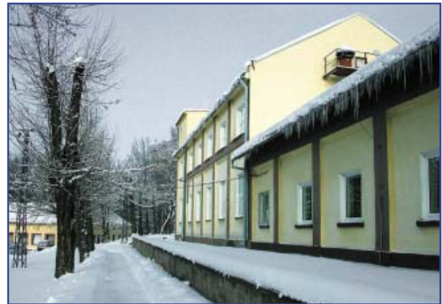
Electrical Plant Building
